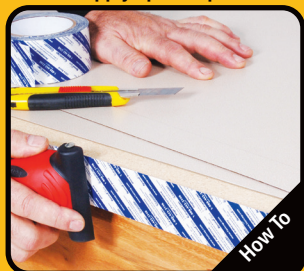
Roll for maximum adhesion
