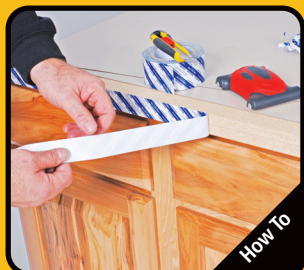
Remove liner, apply edging
